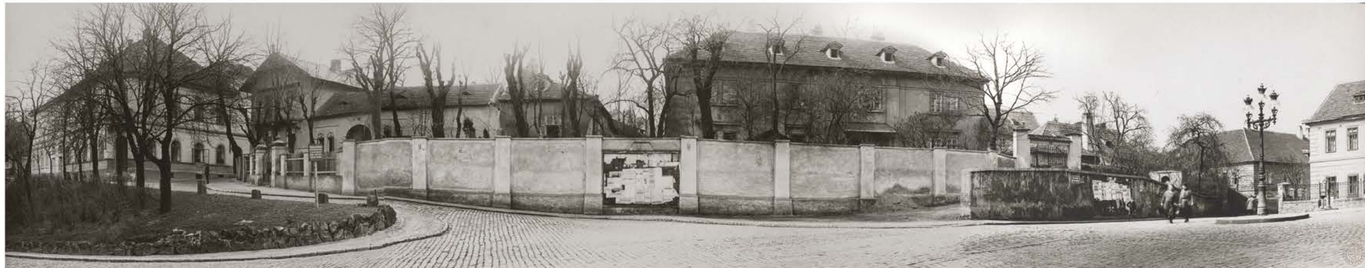
The Bubeneč acropolis. Western side of Kostelní (today Krupkovo) Square. Left to right: nos. 77, 4, 5, 6. All these buildings were demolished in favour of a Russian secondary school around 1975. Photo by Antonin Alexandr, 1925. Prague City Archives
