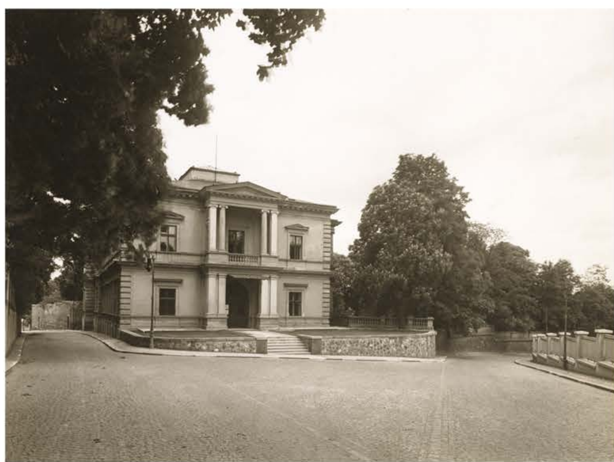
The neighbouring Villa Lanna with its façade between Pelléova and V Sadech Streets is certainly the most famous villa in Bubeneč. It was designed by the architects Antonin Barvitius and Vojtěch Ignác Ulmann in the historicising Neo-Renaissance style. Photo by Trousil, around 1935. Prague City Museum
