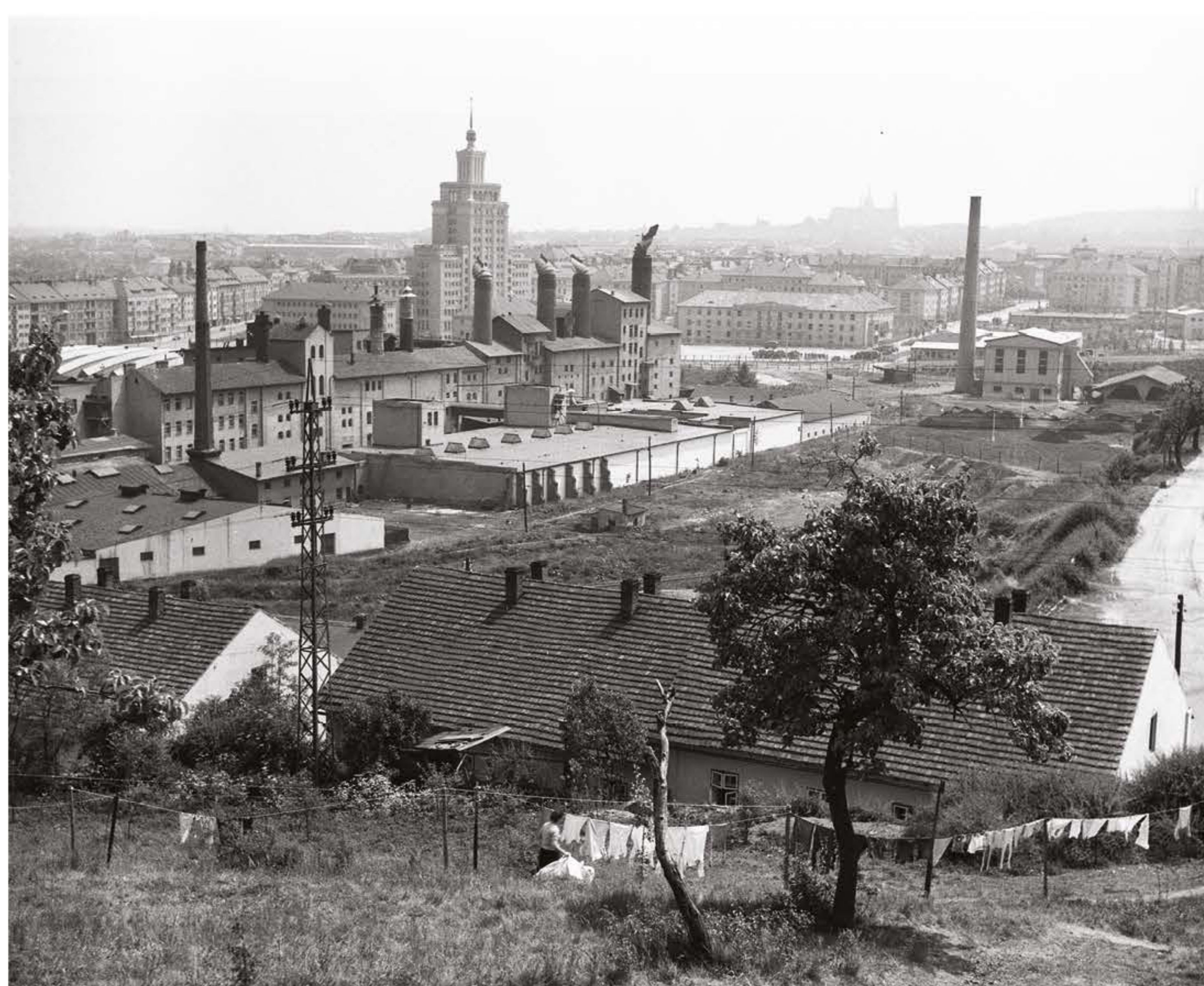
After 1958, Hotel International took up the role of the Podbaba dominant. Today, a residential complex in Patanka Street is situated on the site of the malthouse and its surroundings. Photo by Jan Novotný, around 1960.
