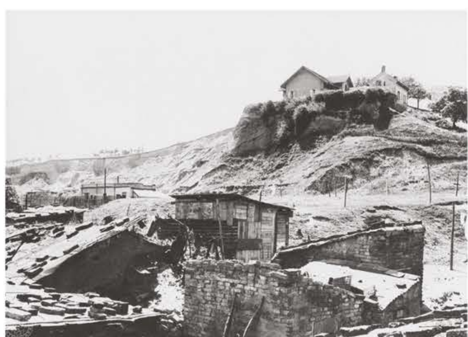
Štáhlavka Homestead no. 27 on a promontory above the brickyard's clay pit. The gradual removal of the slope brought a threat of landslides and other problems. The operation of local brickyards was discontinued only during the Second World War. Photo by Antonín Alexander, 1925. Prague City Archives
